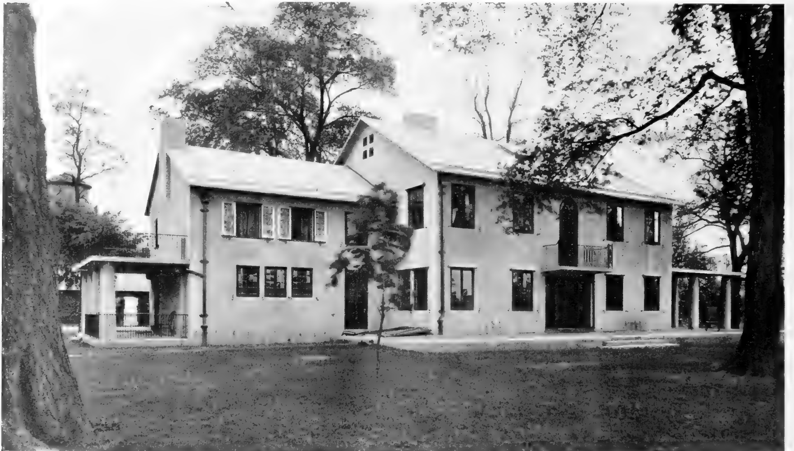
4—The House, Showing the Roof of Reinforced Concrete. The Kitchen Extension and the Servants' Porch are Excellent Features of the House
